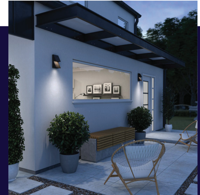
Sconce lights provide a concealed source of light and an ambient lighting effect for outdoor areas in the evening while preventing light trespass onto other properties.
