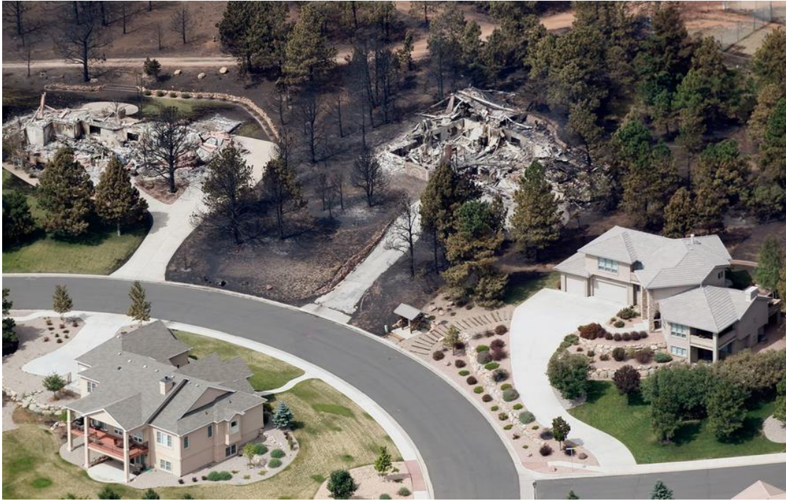
Waldo Canyon neighborhood destroyed by embers.
