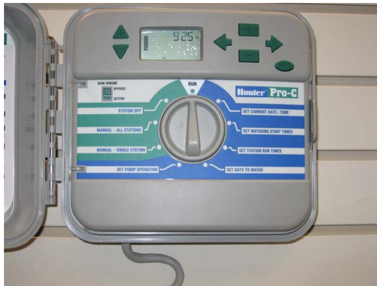
Automatic Sprinkler Fixture (Photo: Dick Bartholomay)
